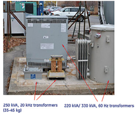
Fig. 5. High frequency vs line frequency transformers.
